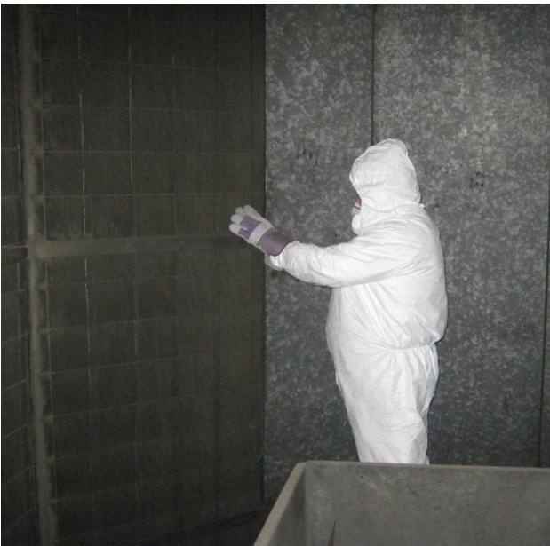
Image 2—Inspection of fresh air filters in War Memorial Offices
