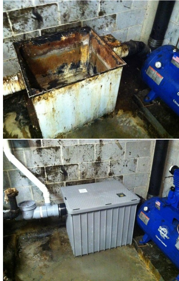
Image 3—Before and after grease trap replacement at Law Enforcement Training Academy
